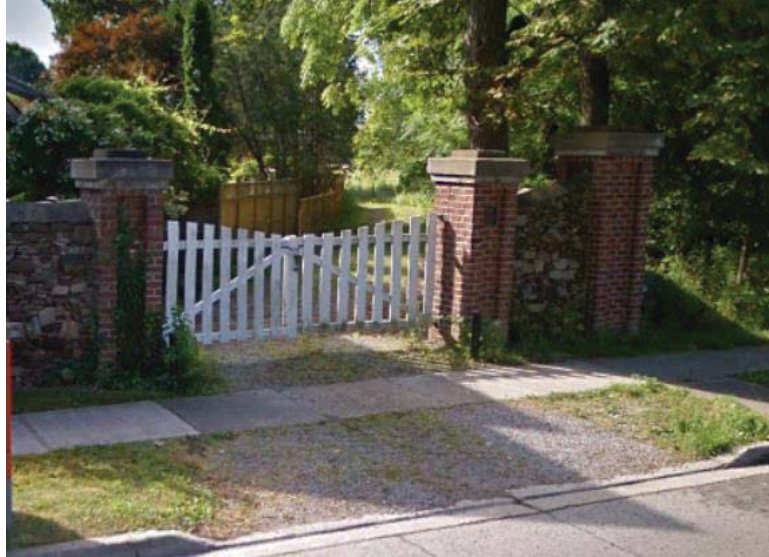
Figure 3: Existing Access to Charlotte Street
