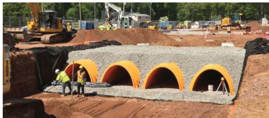
Figure 7: Example Open-Bottom Arch Chamber System
